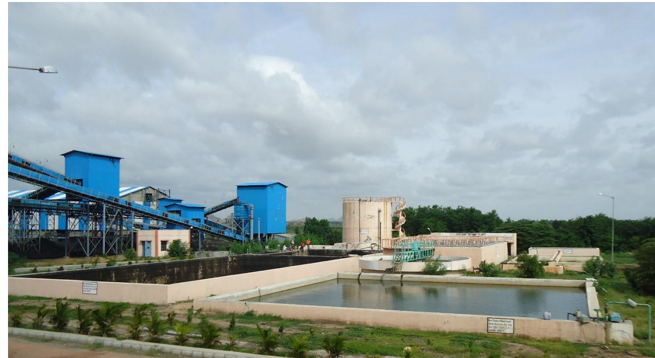
Picture 7: Wastewater treatment plant anaerobic system followed by aerobic system
